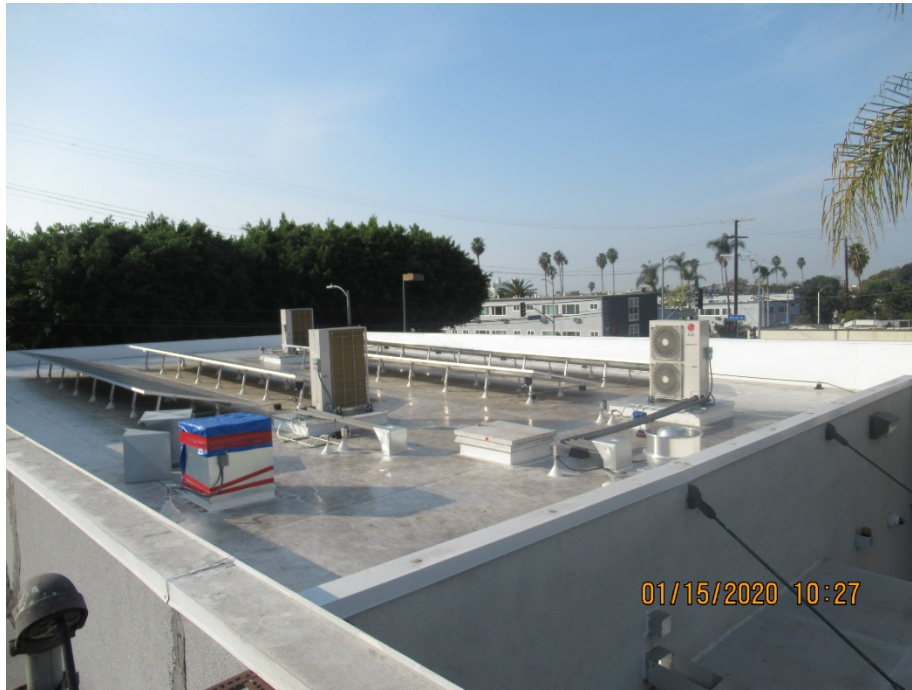
5. Roof of adjacent office property to the west.
