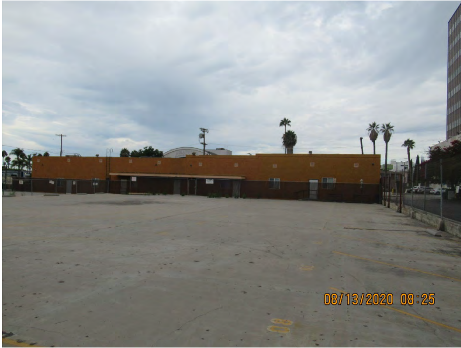
9. Eastern elevation of subject building and rear parking area.
