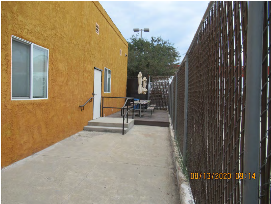
17. Small patio area on the eastern elevation of the subject building.
