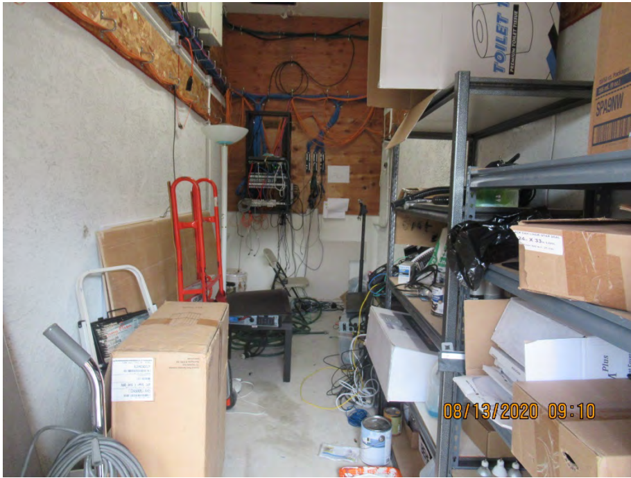
15. Exterior storage space.
