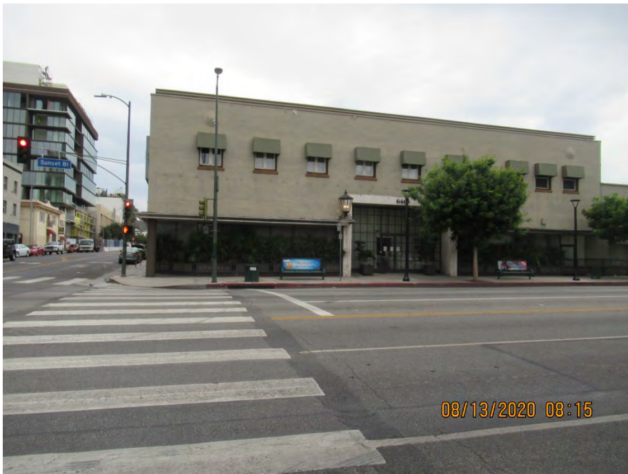
2. Adjacent properties looking across Sunset Boulevard to the north.
