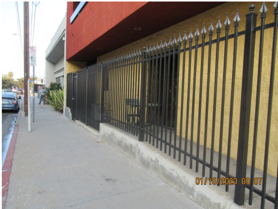
6. Southern elevation of the subject building facing De Longpre.
