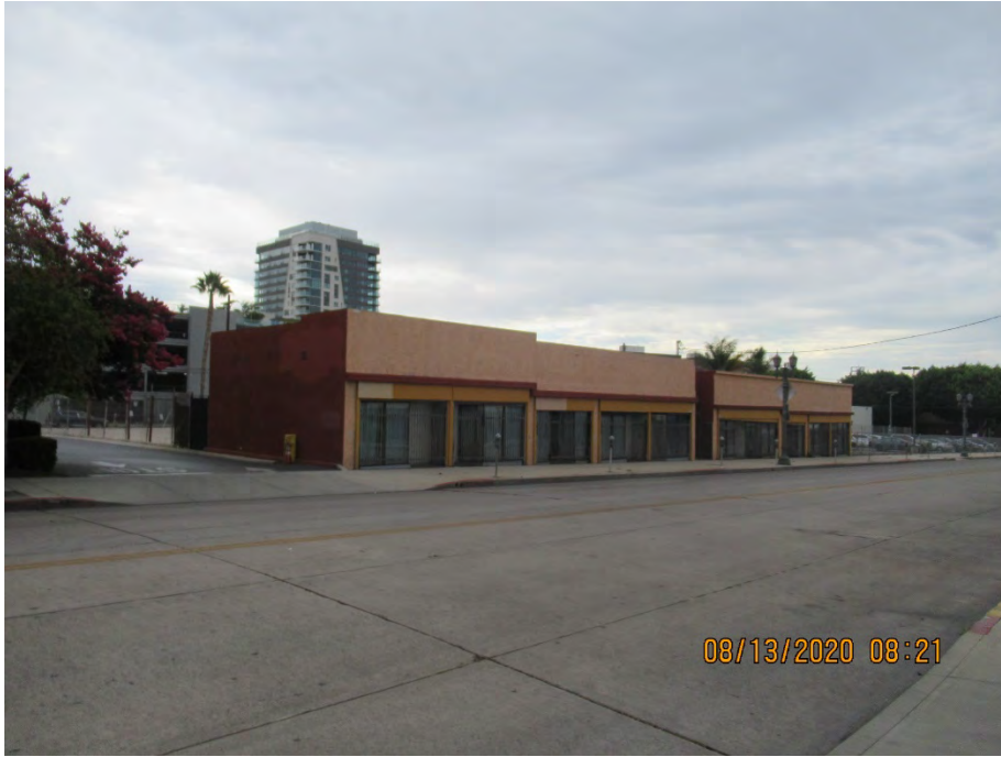
1. View of subject property looking from Wilcox Avenue to the east.
