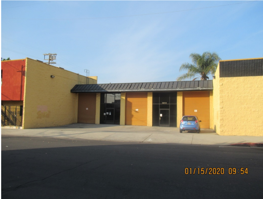
1. Subject building looking across Cole Place to the west.
